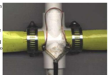
Figure 1 shows the method used to attach the driven element to the PVC cross.
